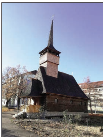
Fig. 1. The historic monument wooden church, University of Oradea, Campus, photo December 2018
